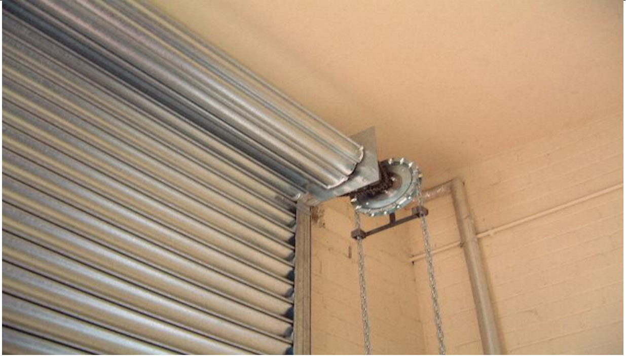
Figure 3 RSD CHAIN OPERATION
